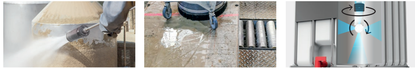
General gun blasting work Surface cleaning
